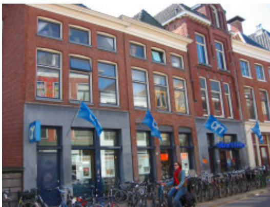
Figure 24: An example of adaptive reuse where three contiguous buildings were remodeled to integrate the interiors and accommodate an Albert Heijn departmental store
